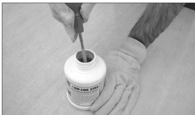
8. Stir solvent cement.
