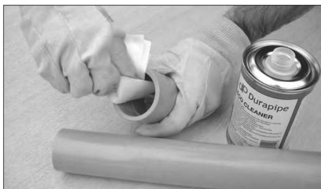
7. Clean pipe and fitting with eco cleaner.
