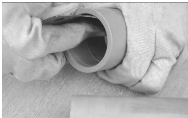
4. Abrade pipe and fitting.
