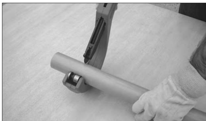
2. Cut pipe to required length.
