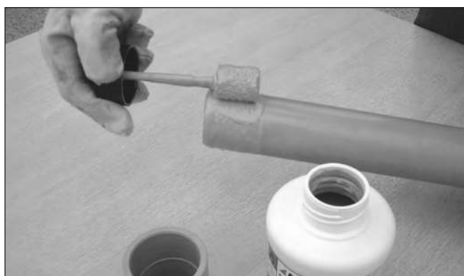
9. Apply cement to pipe and fitting.
